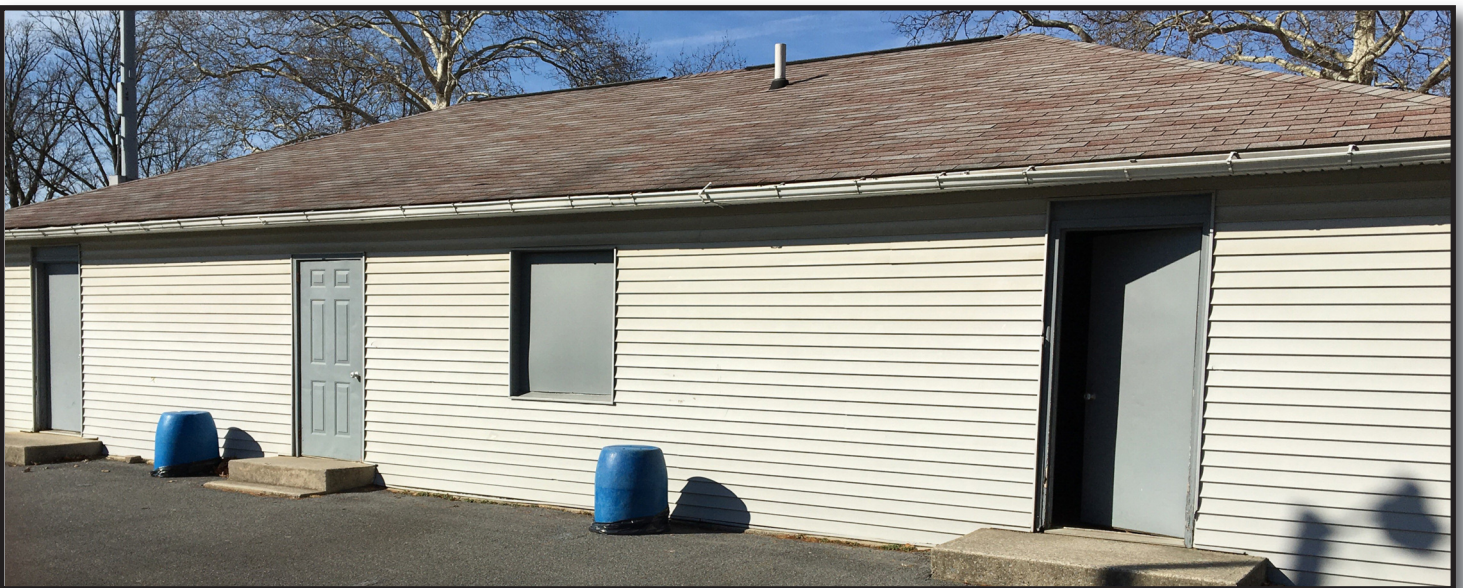
Existing locker rooms
